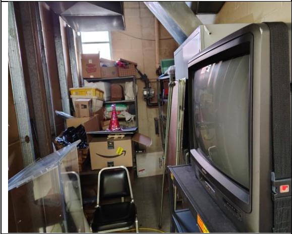
Overview of Room 3 Storage/Mechanical Room
