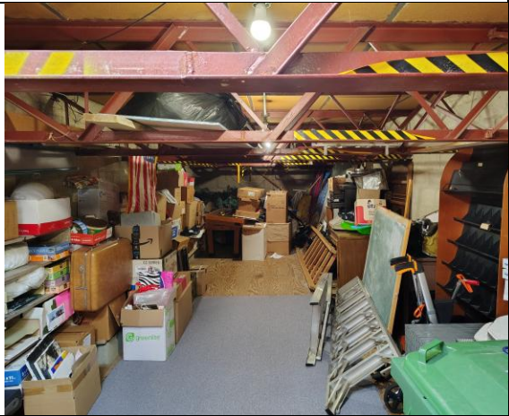
Overview of Room 27 Storage – Second Floor
