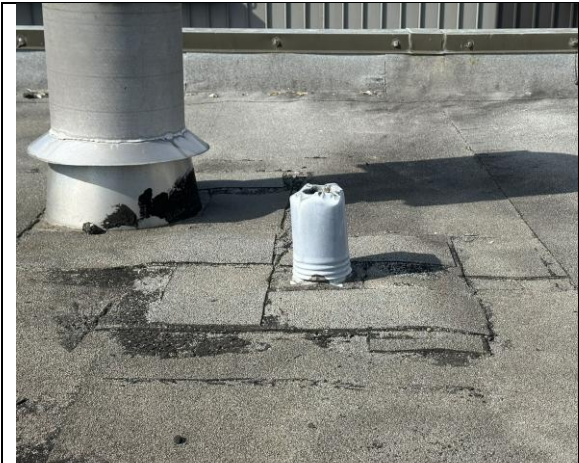
Reading #7 - Roof Pipe Lead Pipe
