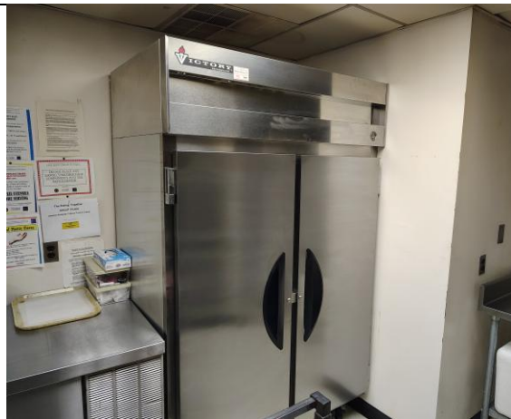
Representative Commercial Refrigerator Assumed ODS-Containing Equipment
