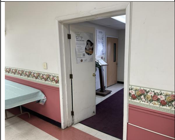
Reading #27 - White Door Frame Lead Based Paint
