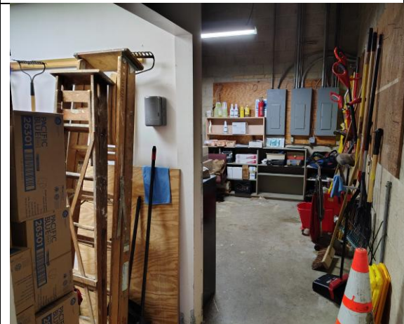
Overview of Room 18 Janitor Storage
