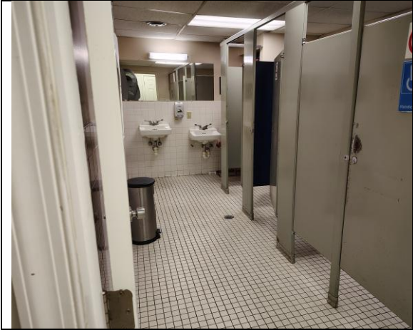
Overview of Room 19 Women's Restroom
