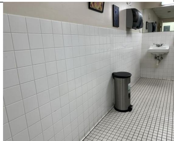
Readings #84 & 85 - White Ceramic Tile Lead in Glazing
