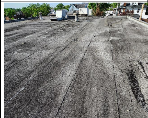
Overview of Roof Upper Level
