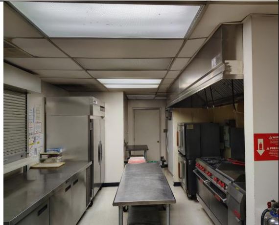
Overview of Room 23 Kitchen
