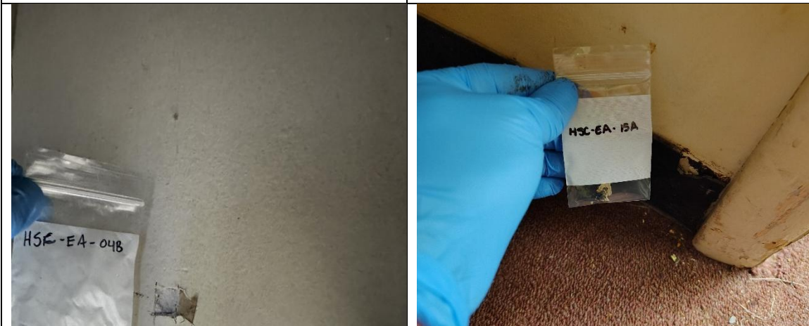
Joint Compound ACM – 2% Chrysotile
