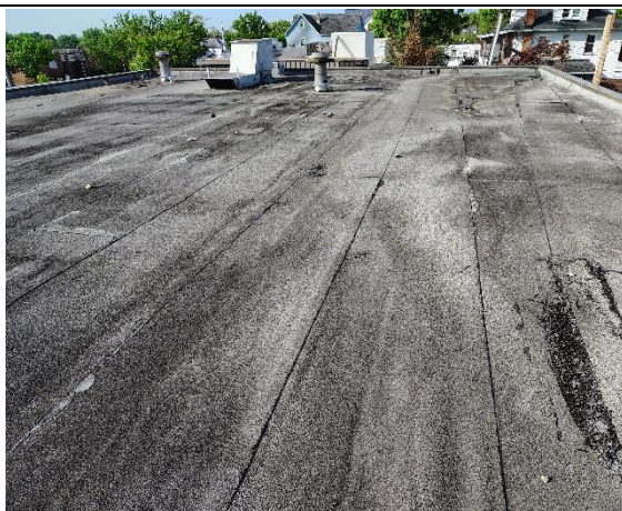
Overview of Roof Upper Level
