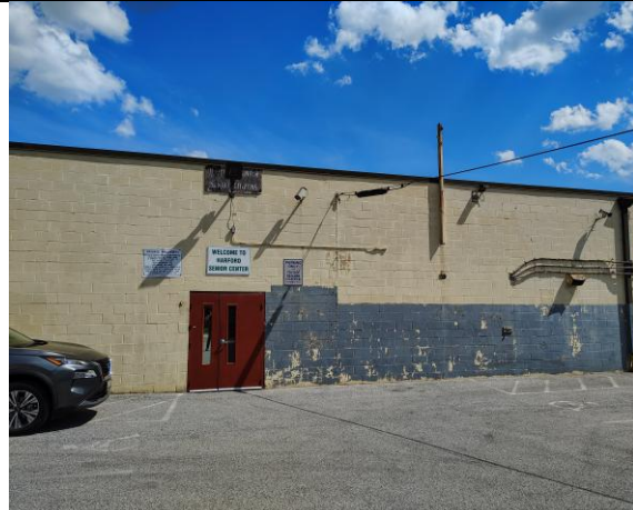
Harford Senior Center Rear of Building
