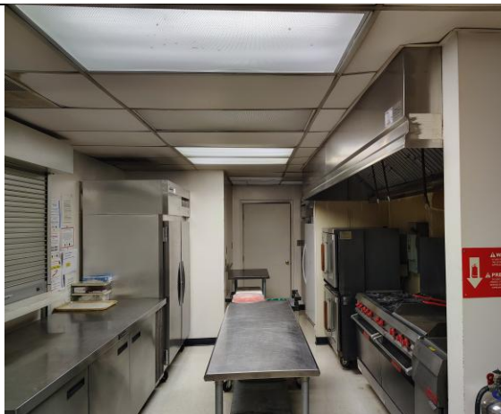
Overview of Room 23 Kitchen
