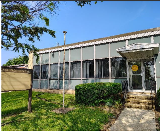
Harford Senior Center Front of Building
