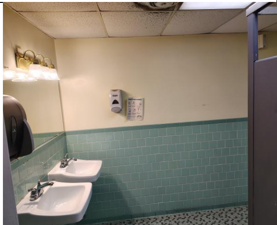
Overview of Room 24 Men's Restroom
