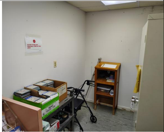
Overview of Room 9 Storage
