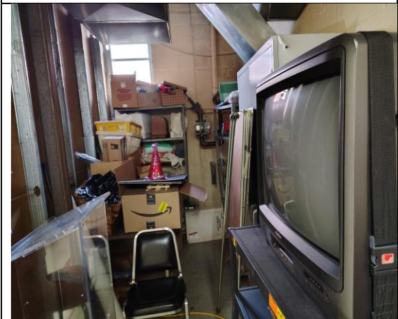
Overview of Room 3 Storage/Mechanical Room
