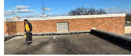
Image 6: Structurally Restricted Louver Sill
